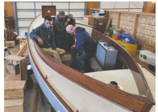
Team Rosinante prepare for propulsion battery installation.
